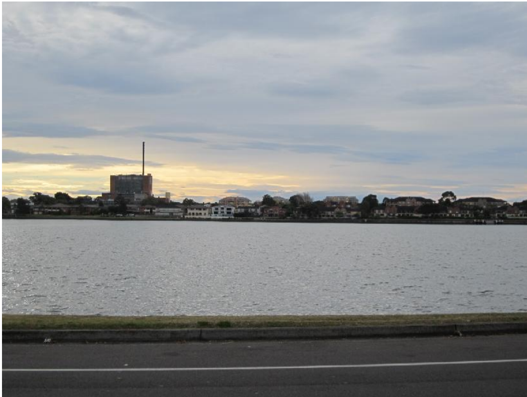
View of the site from Lyons Road West
